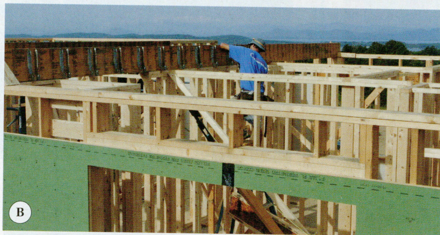
Figure 4. Once the first-floor walls were in place, the crew could install the second-floor support beams (A). While many of the beams were precut (B), a large 5 \frac{1}{4} -inch-wide by 24-inch-deep by 28-foot-long beam built up from three 1 \frac{3}{4} -inch by 24-inch LVLs was not, which allowed the crew to verify the length of the span, then cut and fit the beam one ply at a time (C).
