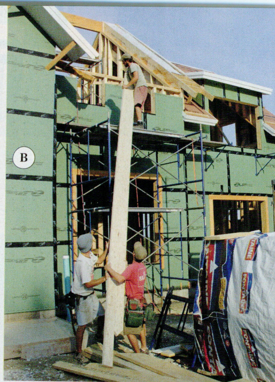
Figure 7. Some of the common rafters had to be cut on site from stock material (A). LSLs are a lot heavier than I-joists or sawn lumber; wrestling the 20-foot-long common rafters into position was a three-man job (B). Crew members tacked the dense material in place with a nail gun (C), then used impact drivers to drive structural screws into the framing.
