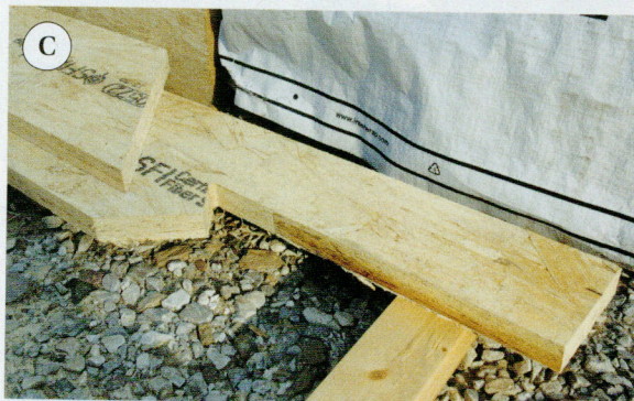
Figure 2. The engineered framing stock is cut with CNC equipment that can accurately trim I-joists and LVLs to length and cut bevels (A). The machine can also cut rafter-tail profiles and make hvac cutouts (B, C).
